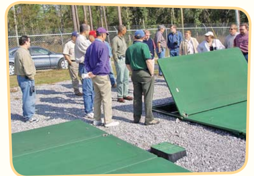
Attendees view decentralized onsite system
